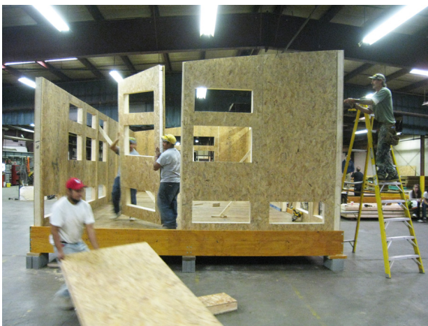
Figure 4. Prototype panelized wall assembly timing
